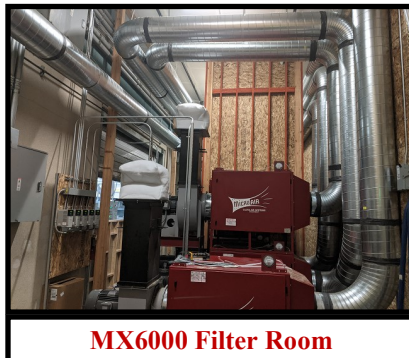
Cyclone Room for Chip Drop-Out
