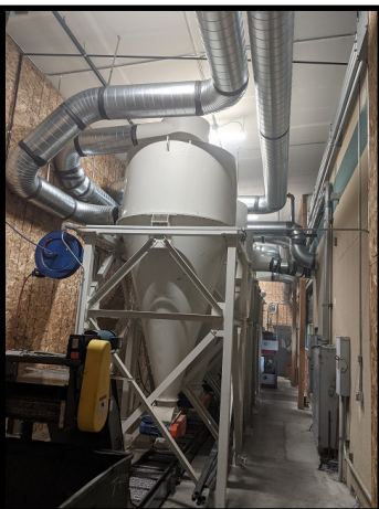
Cyclone Room for Chip Drop-Out
